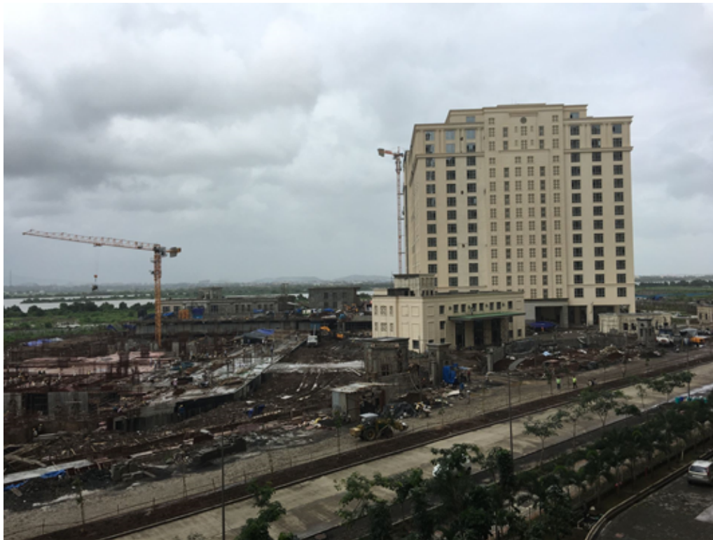
Figure 38: Photograph of the nearly completed TCS building and adjacent developments
