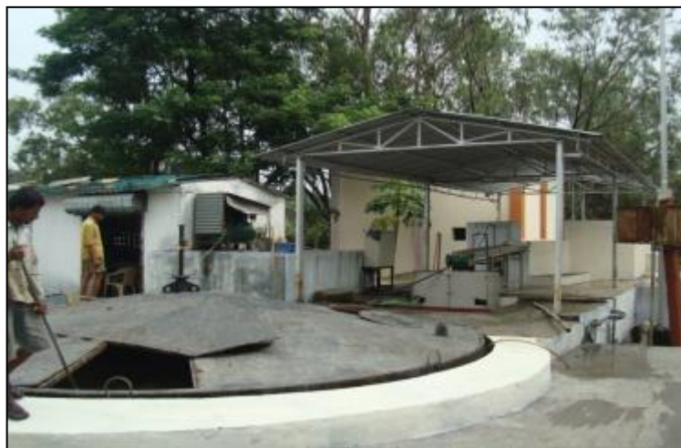
Figure 50: Bio-Methanation Plant at Chhatrapati Shivaji Maharaj Hospital
