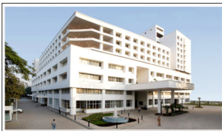
Figure 28: Photograph of the Jupiter Hospital Building in Thane
