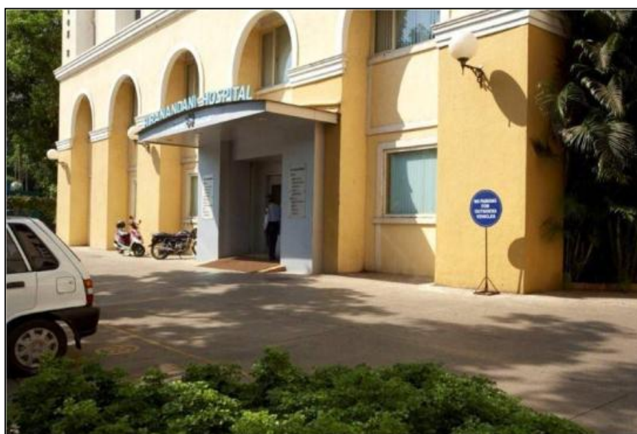
Figure 37: Photograph of the Hiranandani Multispecialty Hospital
